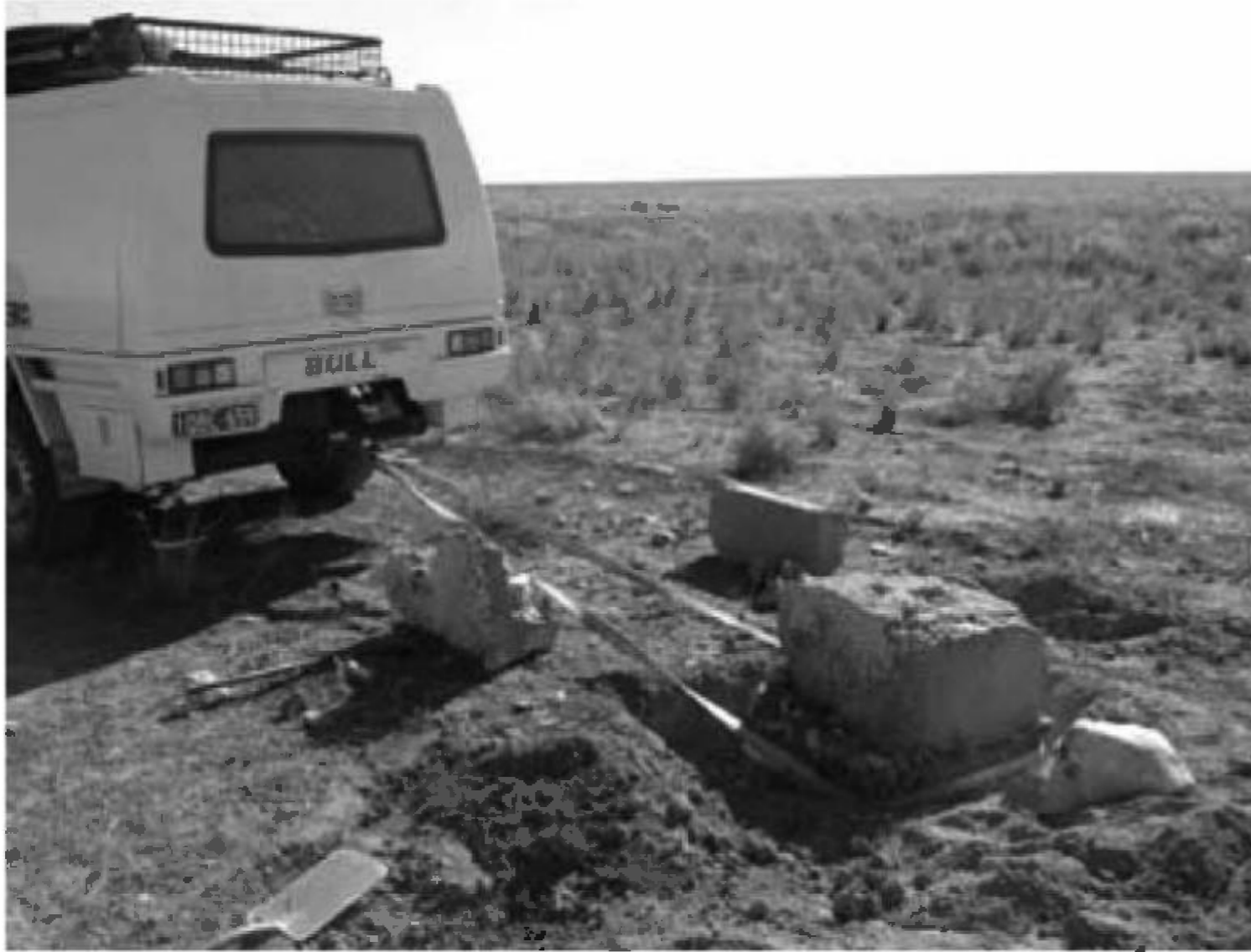
Figure 5. The remains of the Western Deakin astronomy pillar being repositioned back in its original position by Landgate Geodetic Surveyors and Curtin University Survey Students in 2012
